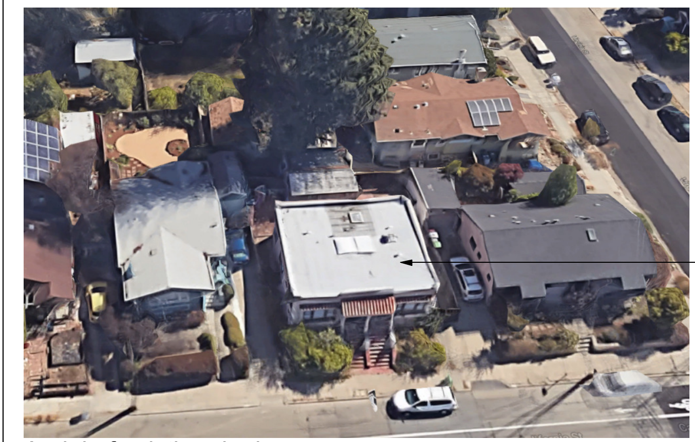
Aerial of existing duplex
